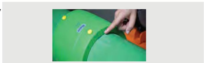
**2.6** Place the pipe fittings on a horizontal frame and ensure that they are fixed properly.
